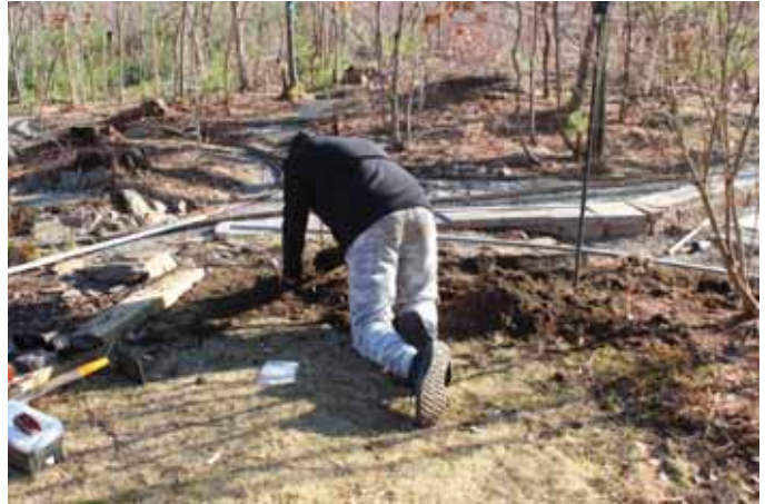
Nephew Trenching for conduit
