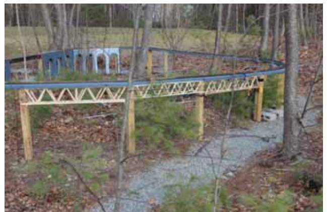
Truss bridges 54, 48, 54 inch.
