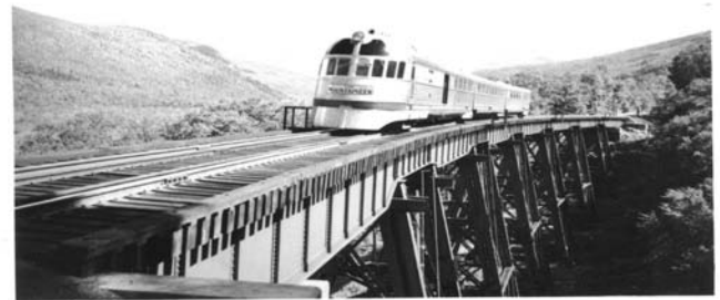
The Mountaineer on the Frankenstein Trestle
