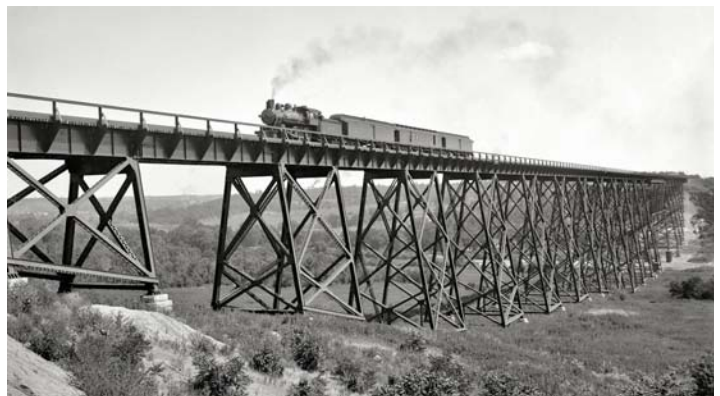
1902 - Iowa Chicago & North Western Railway - Steel viaduct over Des Moines River (William Henry Jackson)
