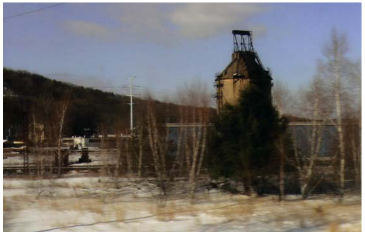
Coaling Tower Cedar Hill Yards, New Haven, CT. This is the former New Haven Railroad freight yard and steam service and maintenance area. East New Haven, CT. 12/27/10
