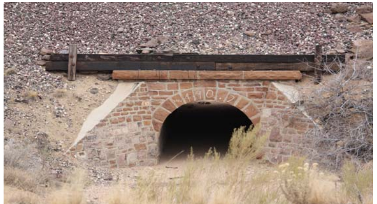
Cut Stone Culvert, MP 490.2
