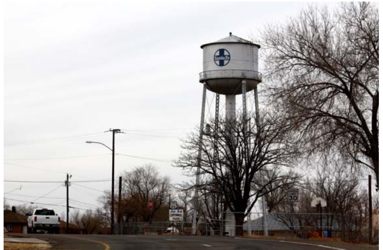
Ash Fork Water Tower
