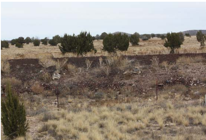
Abandoned AT&SF Roadbed Beside I-40
