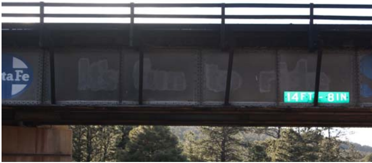
AT&SF Bridge East of Williams on Rt. 66
