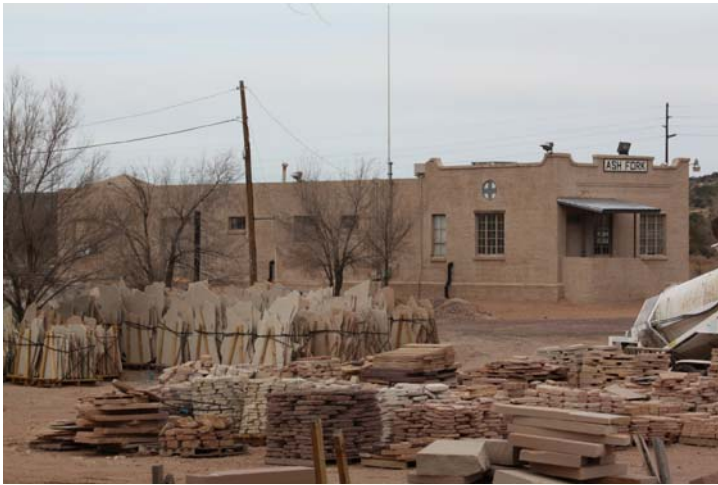
Ash Fork Freight House / MOW Building, Flagstone
