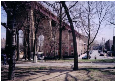
Turning 180 degrees to the southeast shows how the viaduct fits into the residential area of Astoria with the columns towering over the buildings. (Above Photo)
