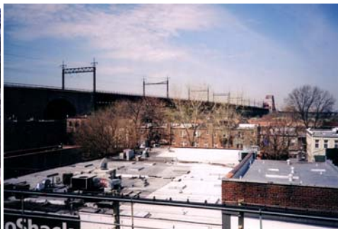
Looking northwest (above Photo) from the platform of the NYC Transit's elevated subway platform at 31st Street & Ditmars Blvd., Astoria, Queens County, NY. The catenary-topped Hells Gate viaduct looms over the residential neighborhood. The Hell Gate Bridge is at the far end of the viaduct.
