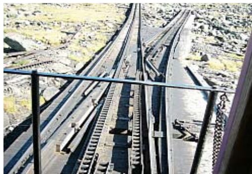
Here is a picture of the old nine-piece switch system still in use at the top passing siding.
